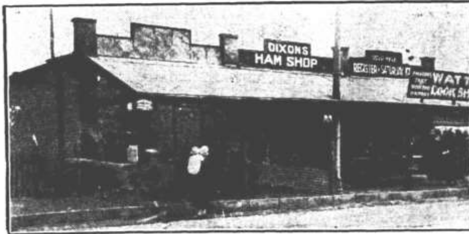
A fire broke out early on Thursday, February 16, in a shop on the Magill road, at Kensington Park North, and completely destroyed the building and its contents. Although the flames spread to the two adjoining shops, causing considerable damage, the Norwood Fire Brigade effected a good save. Damage is estimated at £500.
